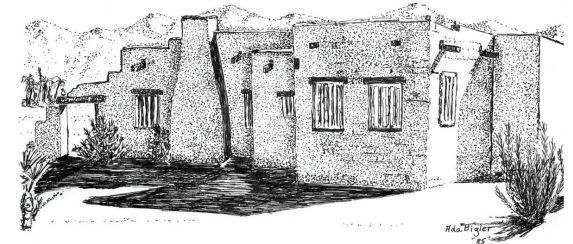
historic adobe gallery at Oasis of Mara
